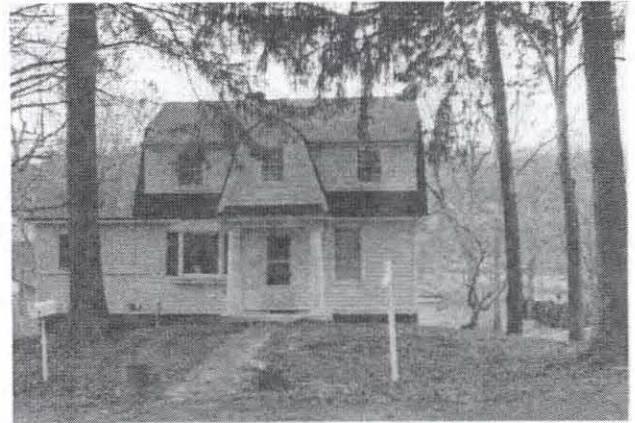
The farmhouse completed
